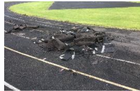
Top Coat Removal
