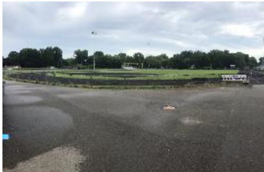
Hilbert Track Replacement
