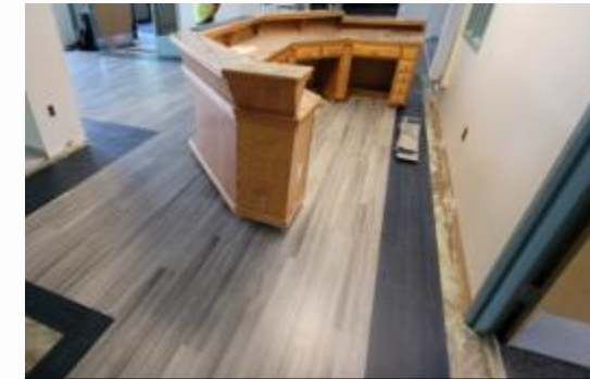
New Flooring Install
