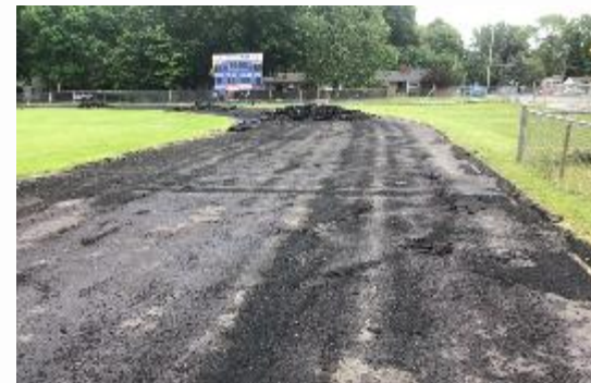
Top Coat Removal
