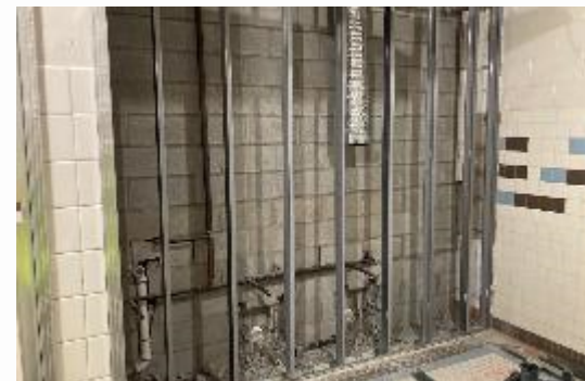
Rebuild of Plumbing Wall
